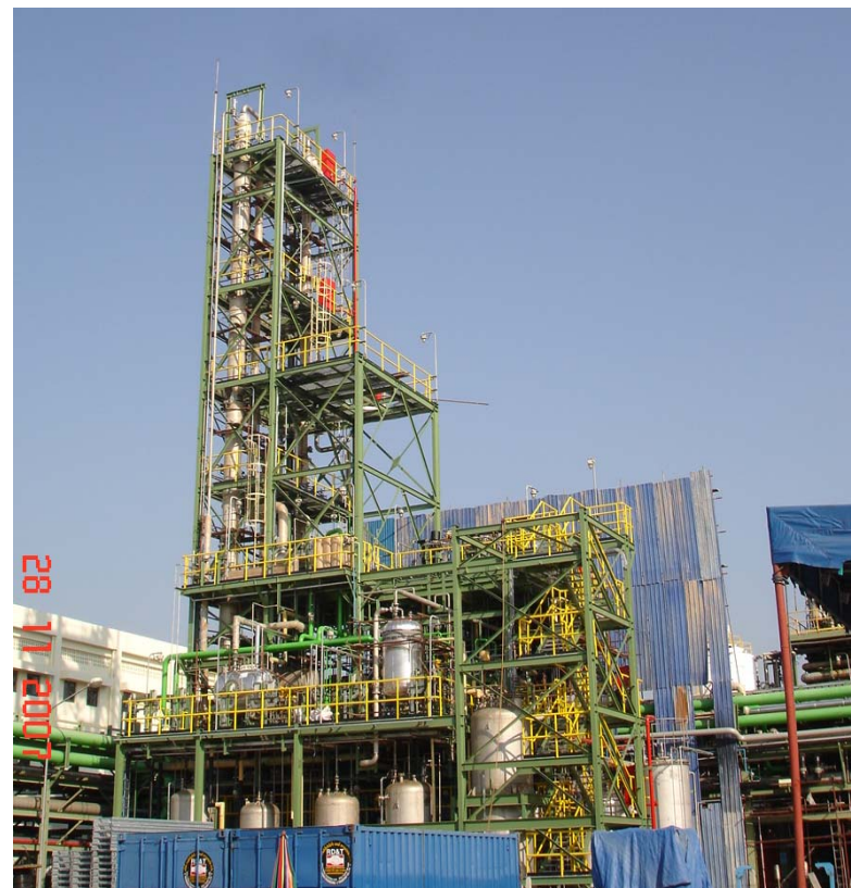
View of 3000 tpa Epichlorohydrin plant at Rayong, Thailand
